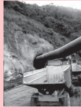
Building an Ethiopian hydroelectric power plant
